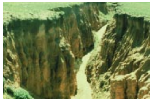
erosion gully, Bredbo, New South Wales (Photo G. Taylor)
