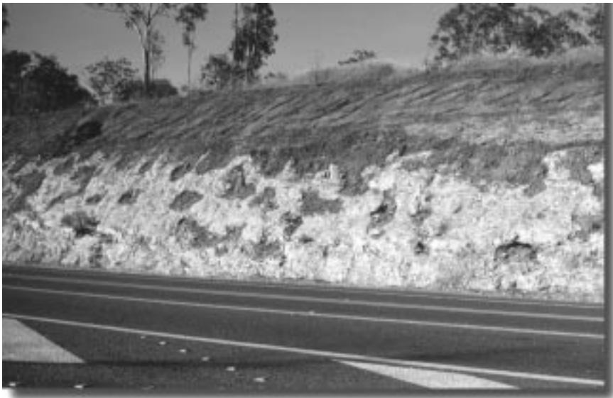
karstic weathering of Cretaceous clay-stone, Tiger Brennan Drive, Dawin, N.T. (Photo R.A. Eggleton)
